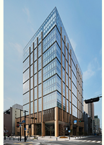
Exterior view of new head office building
